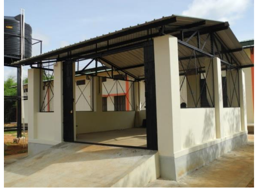
Steam boiler room
